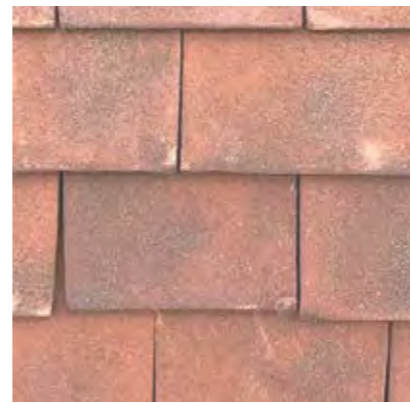
Roof tiles - for Plot 1 and 5 Heritage Clay Tiles Colour: Clayhall Medium Blend or similar approved
