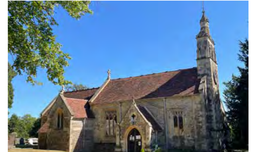
Fig 25 St. Andrews Church (Source: DPDS)
