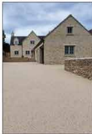
Reference Image: Example of permeable resin bound gravel used for the access way and private driveways/ parking.
