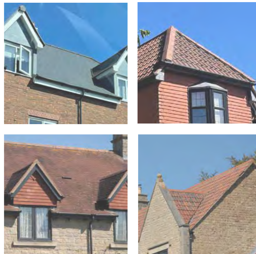
Fig 21 Photos of roof materials found near site for reference (Source: DPDS)
